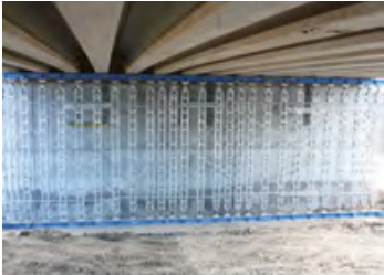
Heavy Duty Shoring
