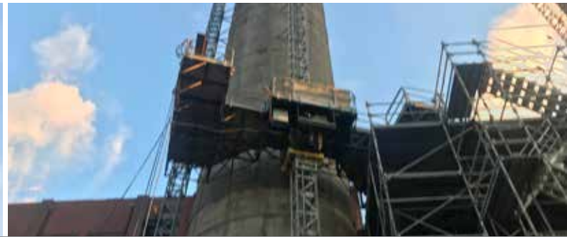
SafRise® Mast Climbers are able to reach heights of over 500 feet with a single-mast capacity of 8,000 pounds. ^
