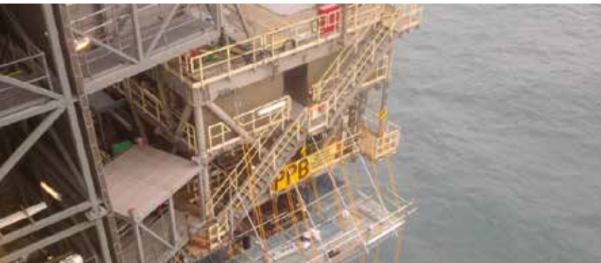
A jack-up rig was positioned beside the platform and integrated via a custom stair tower.
