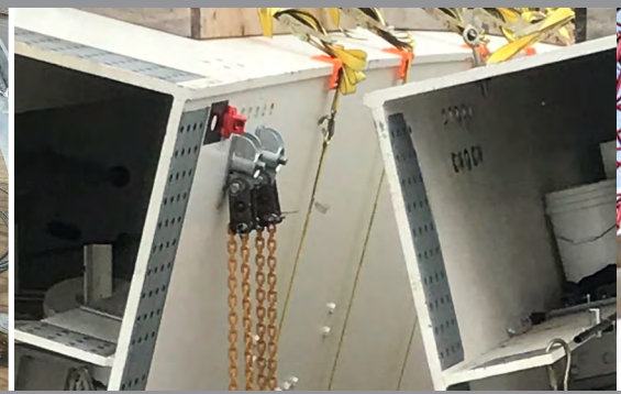
With capacities up to 150 pounds per square foot, built from a few basic modular components and outfitted with guard rails
