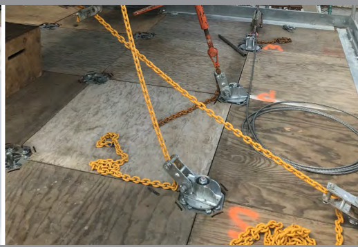
With capacities up to 150 pounds per square foot, built from a few basic modular components and outfitted with guard rails
