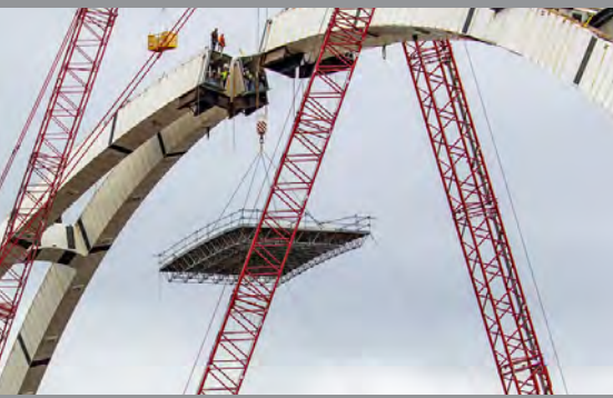
With capacities up to 150 pounds per square foot, built from a few basic modular components and outfitted with guard rails
