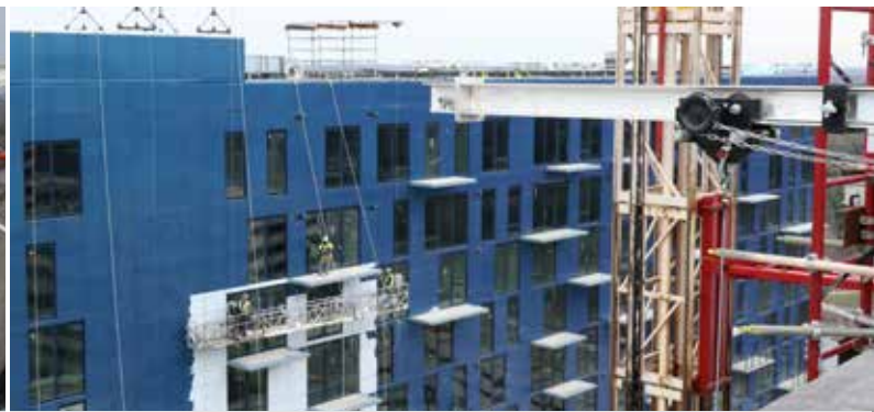
A close-up view of the chain-driven trolley system and the interior end stop.
