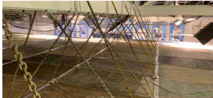
QuikDeck delivered a safe, smooth work surface. ^
