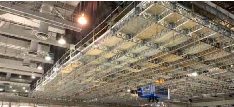
Once pinned, the trusses pivot outward and connect to the next node. ^
