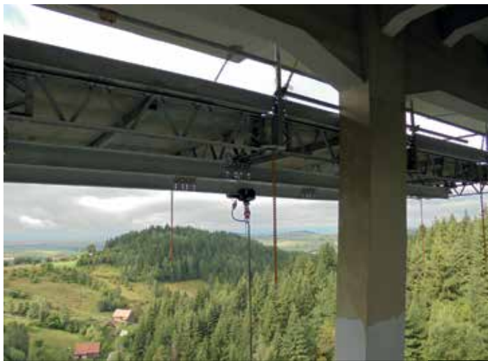
Swing stages were suspended from monorails beneath the platforms
