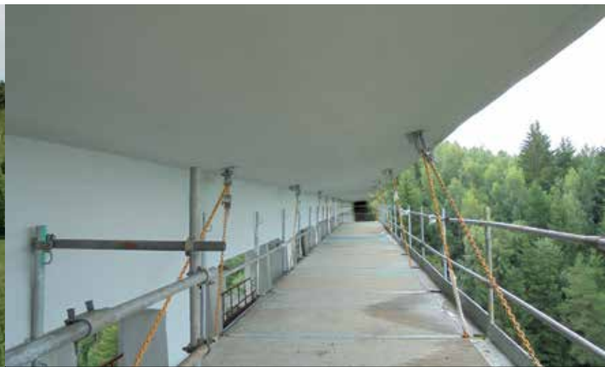
Platforms provided access to the walkway above and the arch below
