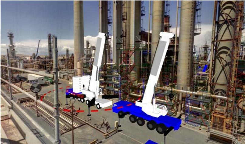
**Figure 4.** Virtual plan for crane locations.
