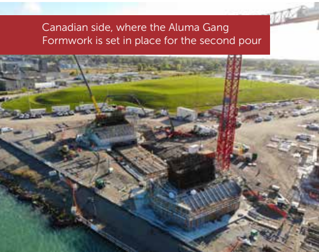
Canadian side, where a pour is in progress for the footings of the A-frame pylons
